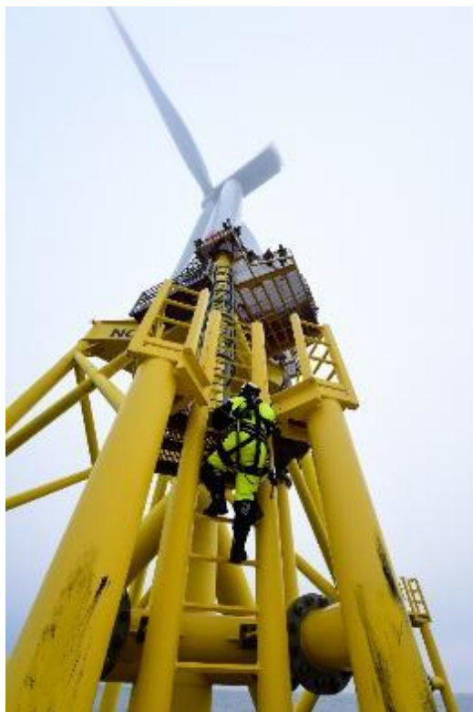
Figure 38 Jacket foundation crew access system and work platform, courtesy of RWE.
