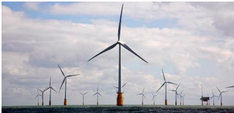
Figure 89 Thanet offshore wind farm, courtesy of Vattenfall.
