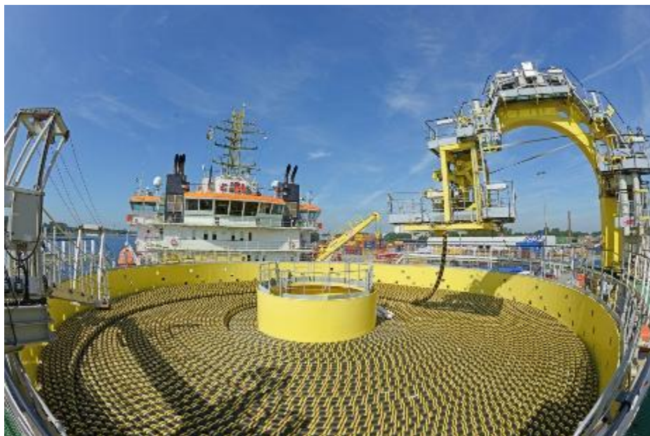
Figure 58 Cable on carousel, courtesy of RWE.
