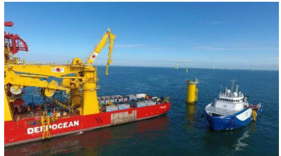
Figure 61 Cable pull-in operations, courtesy of DeepOcean.
