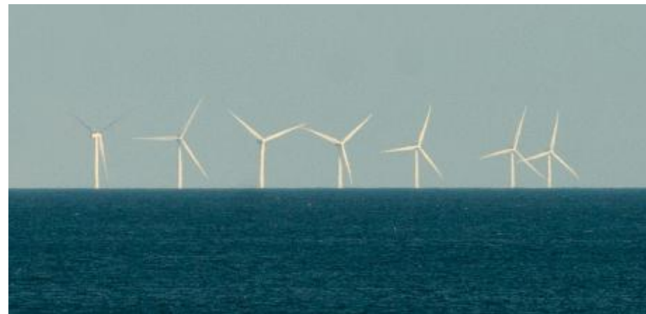
Figure 95 Hornsea Project One wind farm. Creative commons (CC BY-SA 4.0) photo by The joy of all things.
