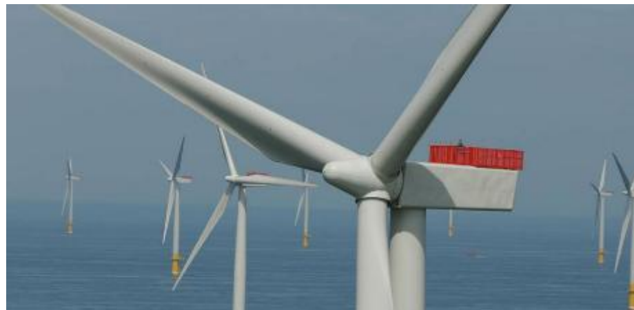
Figure 90 Greater Gabbard offshore wind farm, courtesy of Greater Gabbard Offshore Wind Farm.
