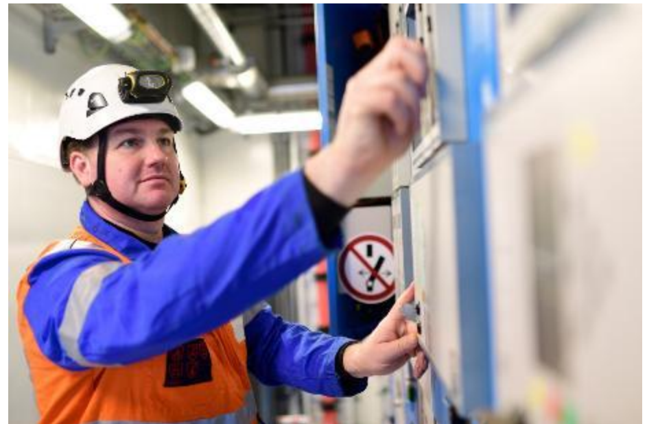
Figure 66 Operative carrying out commissioning works on substation, courtesy of RWE.
