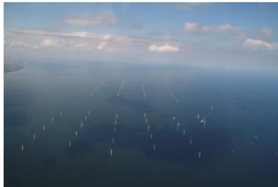
Figure 88 Lynn and Inner Dowsing Wind Farm under construction. Creative Commons (CC BY-2.0), photo by Chris.
