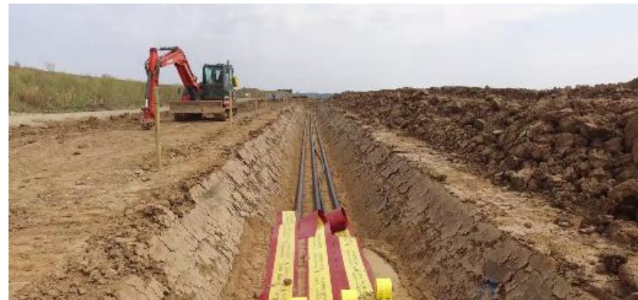
Figure 54 Onshore export cable trenching process. Image courtesy of Ørsted. All rights reserved.
