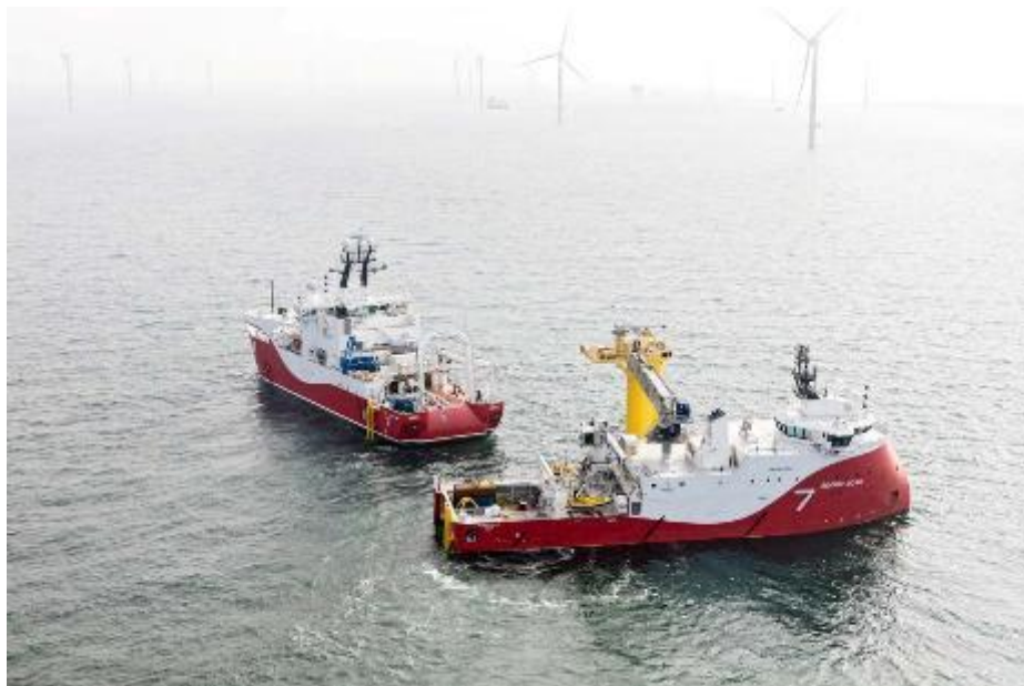
Figure 55 Offshore cable installation works, © Seaway Offshore Cables.
