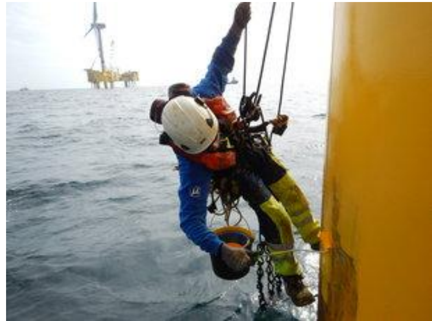
Figure 79 Technicians carrying out foundation inspection and repair works, courtesy of Muehlhan.
