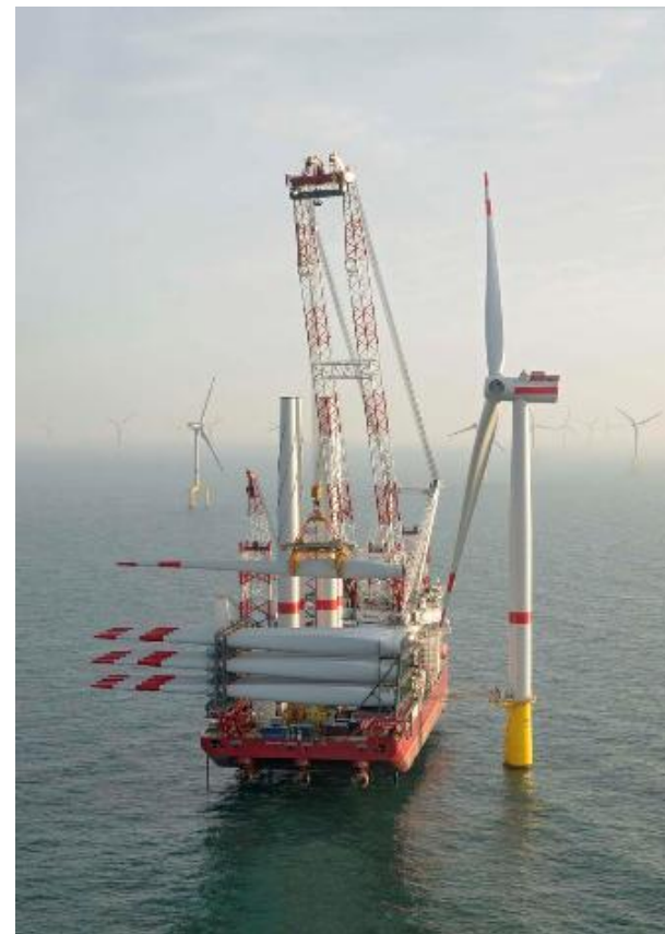
Figure 63 Installation vessel Seajacks Scylla, courtesy of Seajacks.
