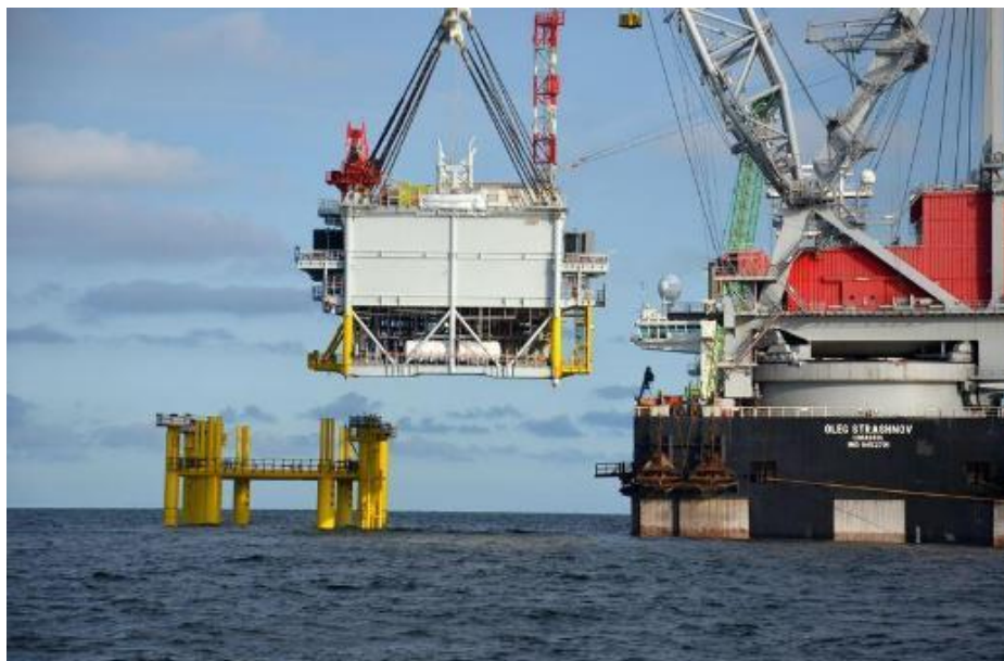
Figure 52 Topside structure of an offshore substation being lifted onto a jacket foundation. Image courtesy of ScottishPower Renewables. All rights reserved.
