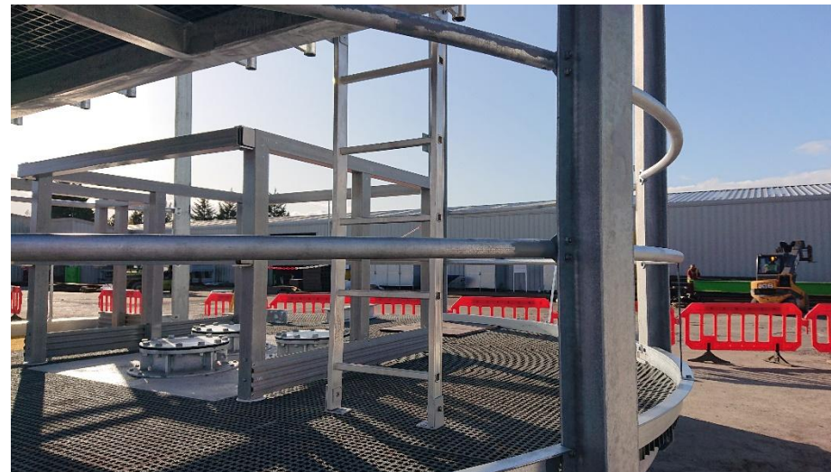
Figure 37 Example of secondary steel, courtesy of Hutchinson.
