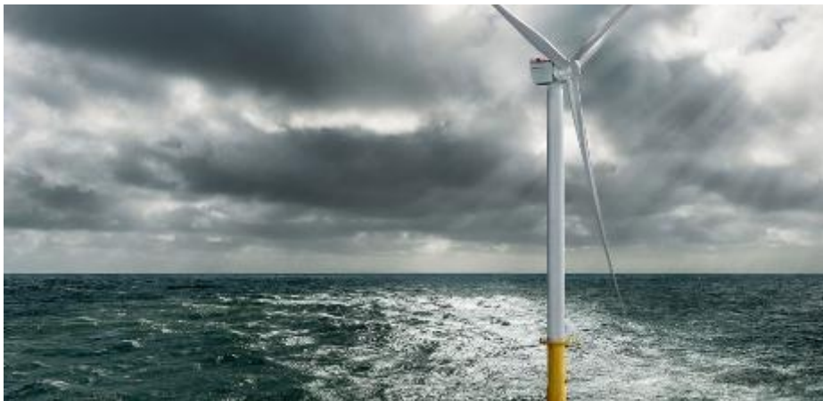
Figure 94 Siemens SG 10.0-193 DD, (c) Siemens Gamesa Renewable Energy.
