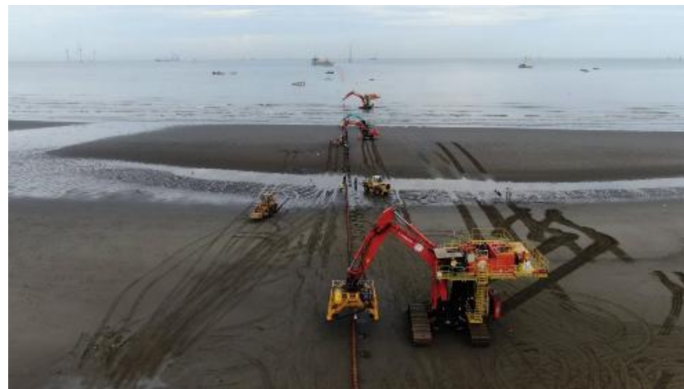
Figure 56 Offshore array cables installed at landfall. Image courtesy of Jan de Nul. All rights reserved.
