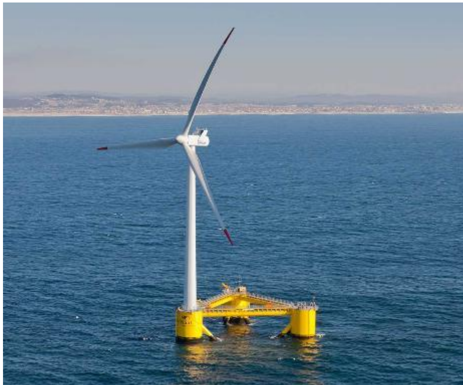
Figure 97 Prototype of the Principle Power floating foundations used in the Kincardine project. Creative Commons (CC BY-SA 3.0) photo by Untrakdrover.
