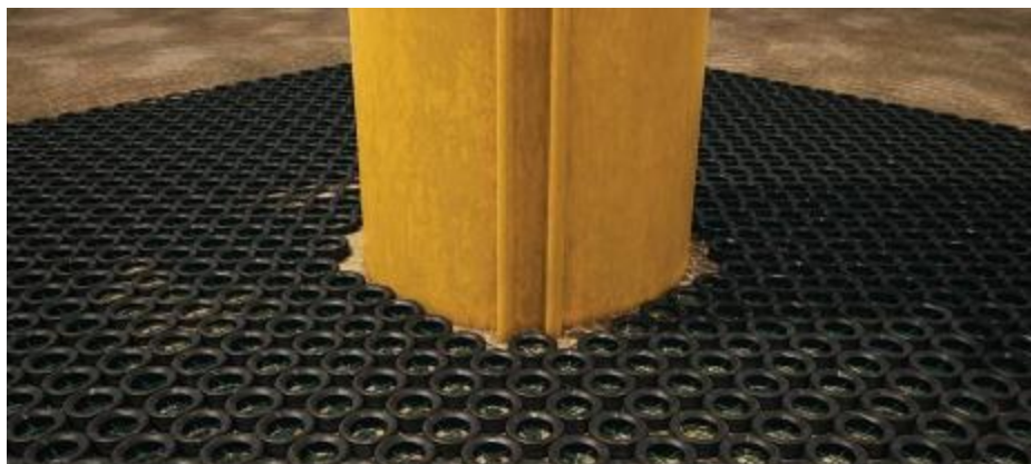
Figure 42 Novel scour protection system visualisation, immediately after installation, courtesy of Scour Prevention Systems.
