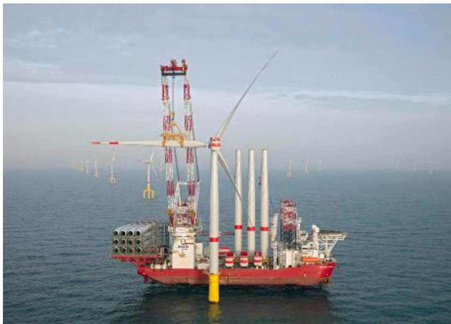
Figure 64 Lifting of third blade during turbine installation, courtesy of Seajacks.
