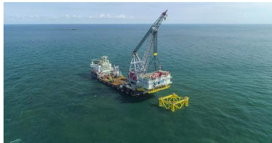
Figure 53 Substation installation vessel, courtesy of ScottishPower Renewables.
