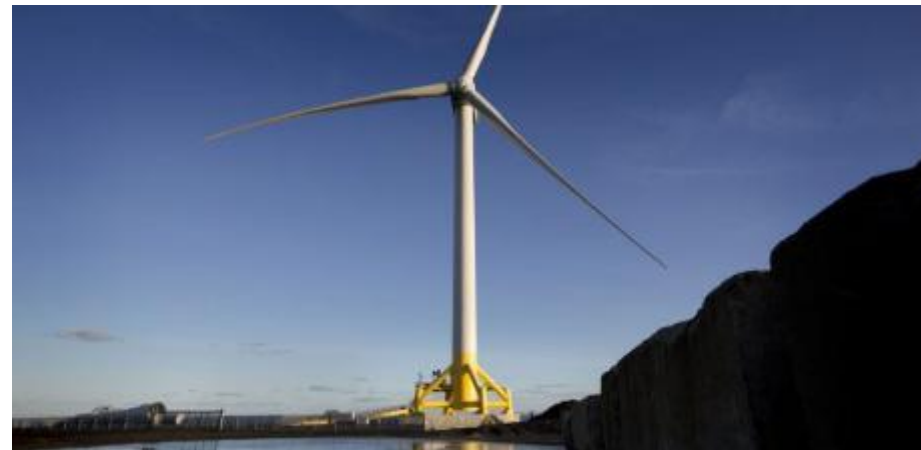
Figure 91 Levenmouth turbine, courtesy of Offshore Renewable Energy Catapult.
