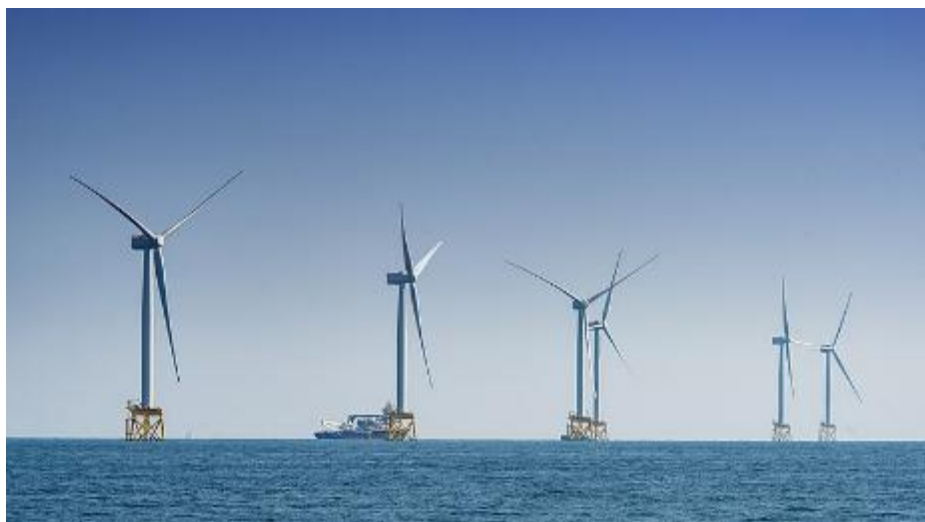
Figure 96 East Anglia ONE under construction, Wikimedia Commons (CC BY-SA 4.0) photo by Trommens
