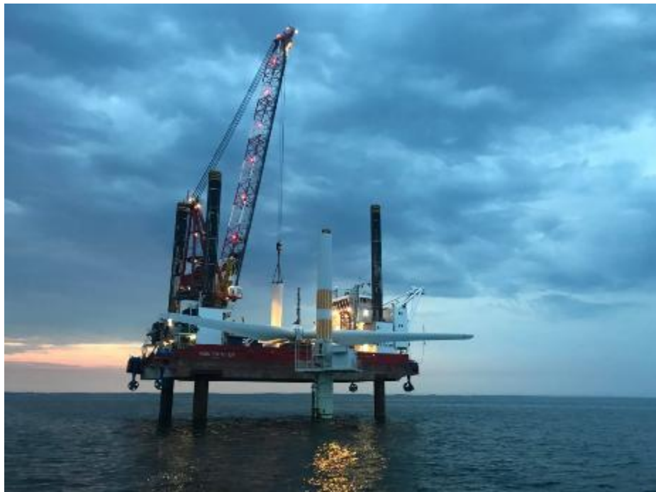
Figure 84 Wind turbine decommissioning operations at Utgrunden offshore wind farm, courtesy of Zitön/Vattenfall.
