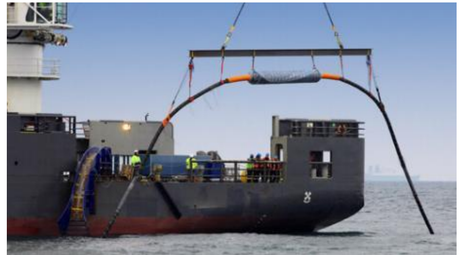
Figure 82 Cable inspection and repair works, courtesy of NKT.
