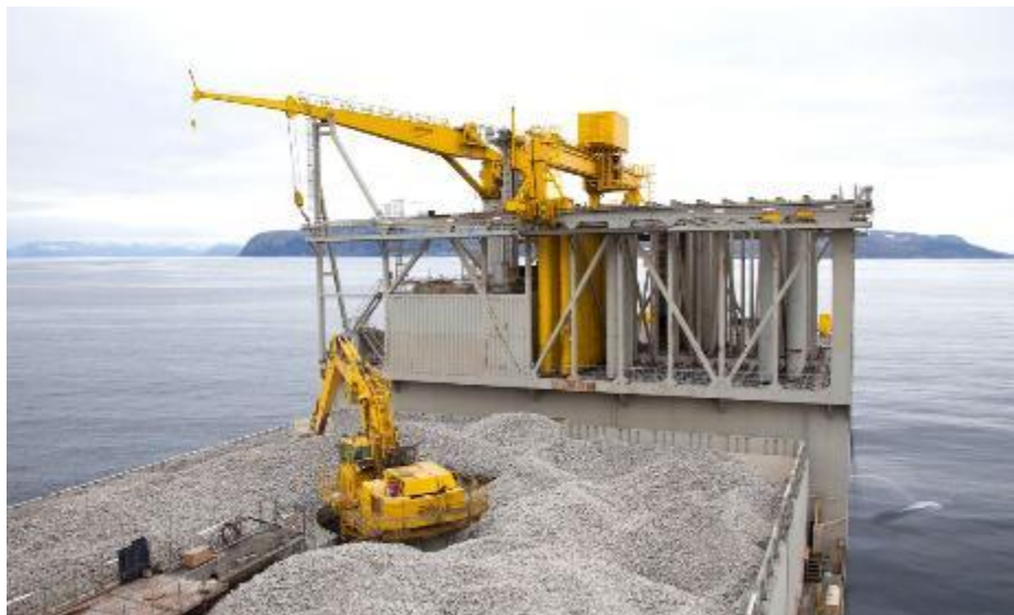
Figure 83 Rock dumping operations, courtesy of Jan de Nul.
